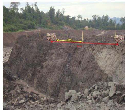
Gambar 4.1.3 Jarak Antar Patok & Antar Batter Pegs
